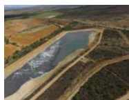
Tailing Management Facility II (TMF II)
