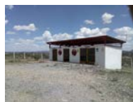
Hazardous waste warehouse.
