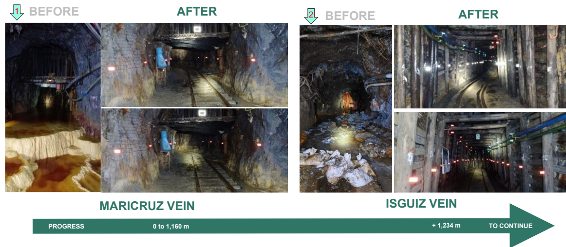
Figure 1: Mine Rehabilitation, Before and After, Level 4090 Click to enlarge
